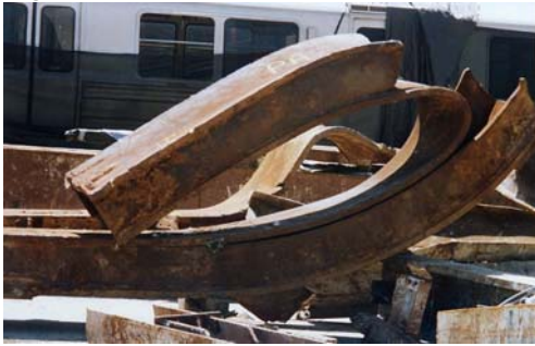
Figure 3. Distorted WTC Steel Beam
